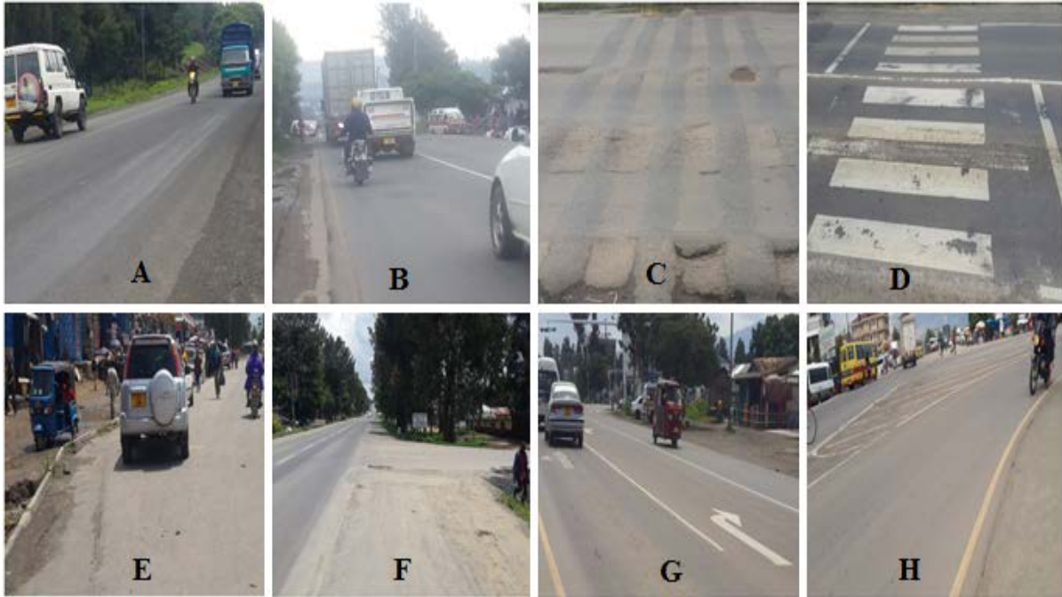
Figure 3.5: Some road markings along Uyole – Iyunga road segment having different disabilities
