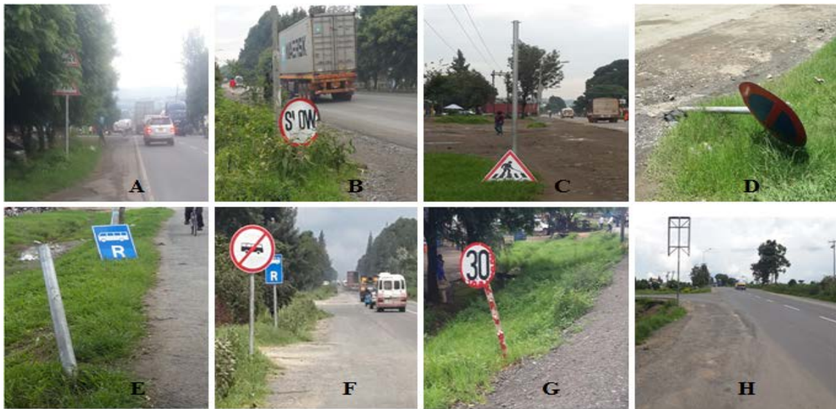
Figure 3.3: Some road signs along Uyole – Iyunga road segment having different disabilities
