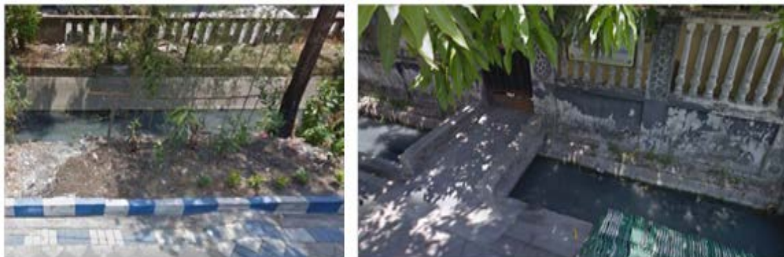
Figure 7: Conditions river/ gutter in Gubeng District
