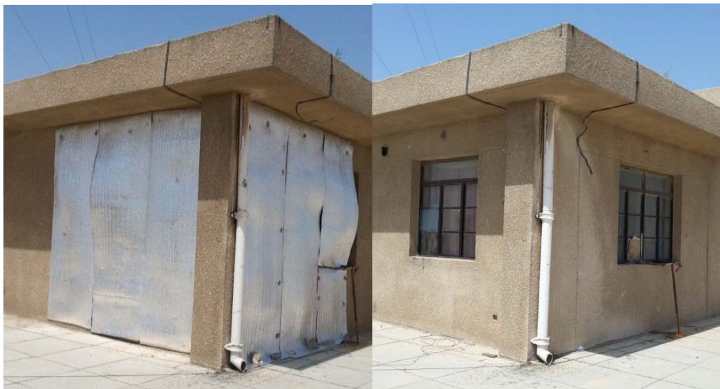
Figure 2: Room before and after insulatin
