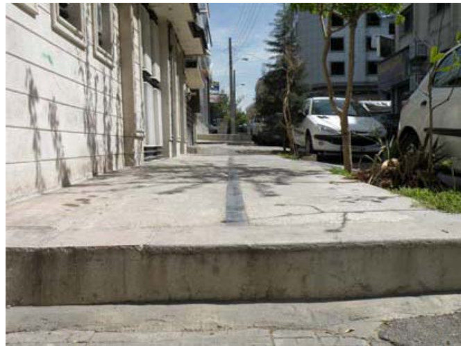
Fig.1. step-shaped connections instead of ramps
