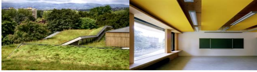
Figure 2: The plant-covered rooftops and its integration with the natural environment in Lyon (on the left) - the floor to ceiling windows and its effect on the natural day lighting in the classrooms (one the right).
