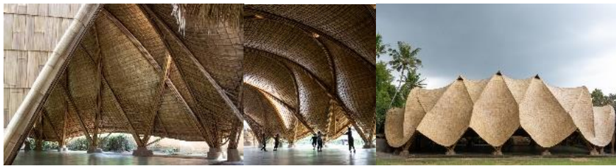
Figure 1: Different views of the bamboo structure of the green school.
