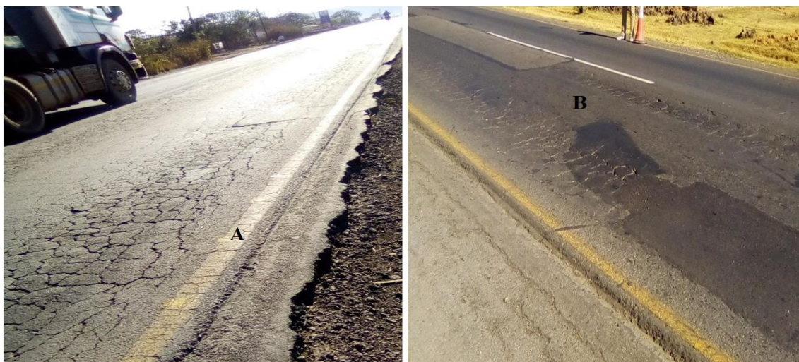
Figure A4: Alligator and edge cracking (left) and alligator cracking and patching (right) for Mbalizi–Ifisi road segment
