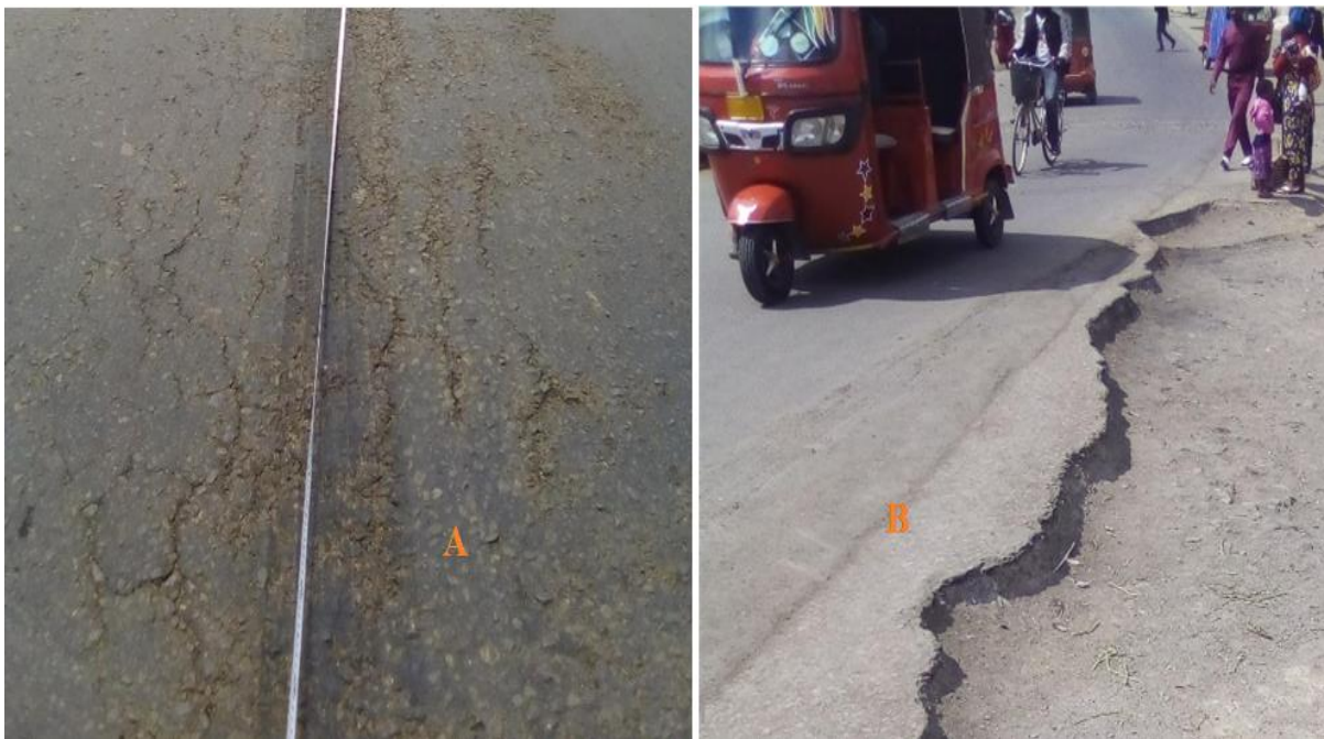
Figure A2: Alligator cracking (left) and edge cracking (right) for Kabwe–Isanga road segment
