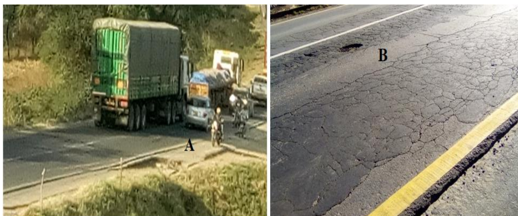
Figure A5: Edge cracking (left) and alligator cracking and pothole (right) for Iwambi–Mbalizi road segment
