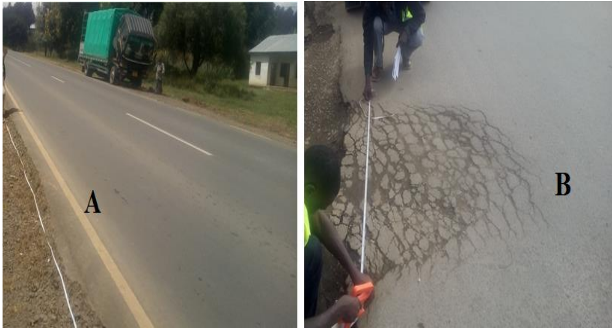
Figure A1: Edge cracking (left) and alligator cracking and edge cracking (right) for Mwahala–Igawilo road segment
