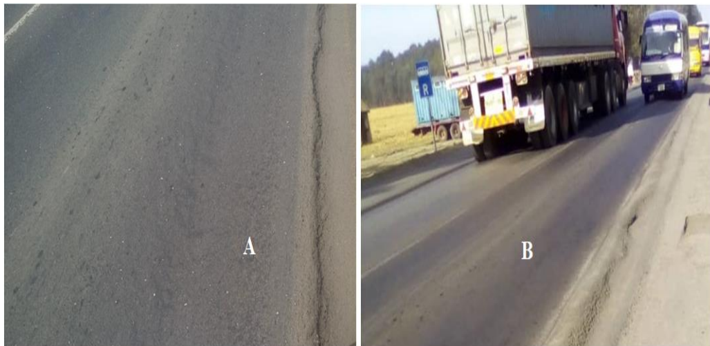
Figure A3: Rutted pavement surface for Nanenane–Uyole road segment
