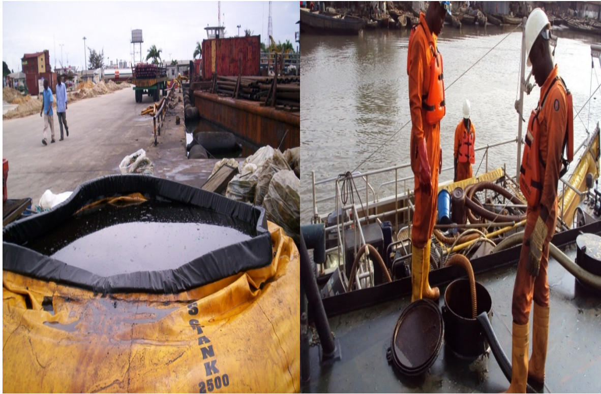
Figure 12&13: Storage and Evacuation of recovered Spilled.
