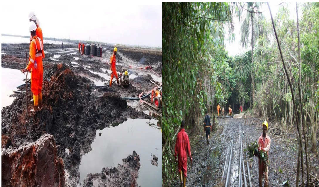
Figure 14 &15: Clean Up and Site Restoration.
