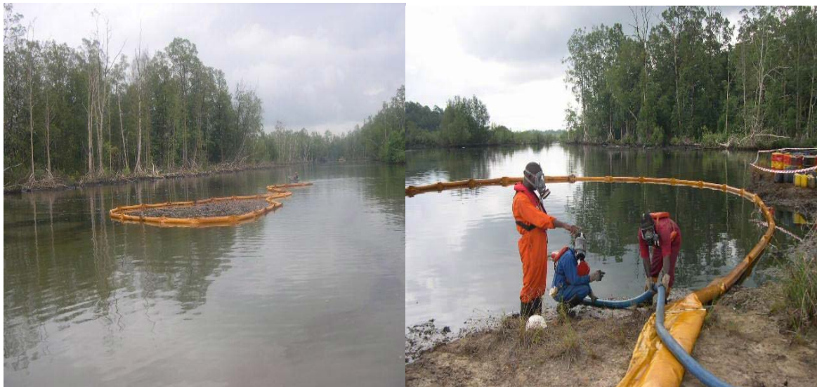
Figure 8&9: Managing Spilled Oil by Boom Corraling.
